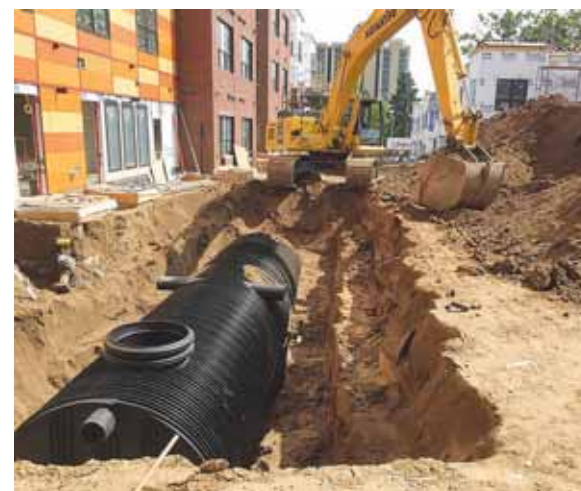
Top: The underground filtration system (left) and storage tank (right) as installation was underway at the Hawthorne Eco-Village Apartments, 617 Lowry Ave. N. Bottom: Some of the Grace Center campus plantings at 1500 6th St. NE. (Photos courtesy of MWMO)
